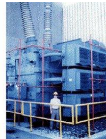
PJM Public Service Step Up Transformer Severe internal damage caused by the space storm of 13 March, 1989
