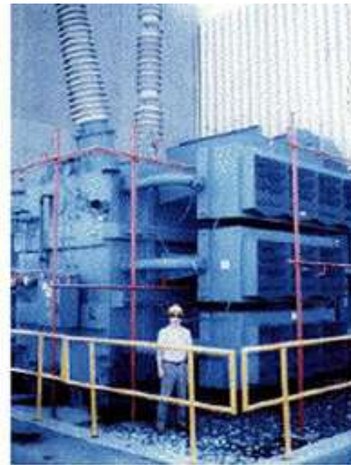
PJM Public Service Step Up Transformer
