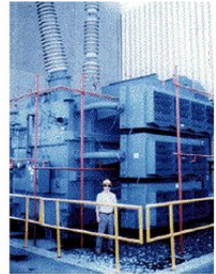
PJM Public Service Step Up Transformer
